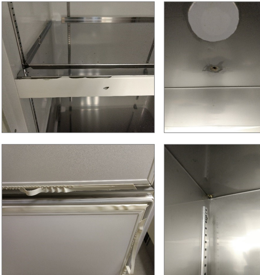
Figure 2. Examples of poor maintenance in freezers
